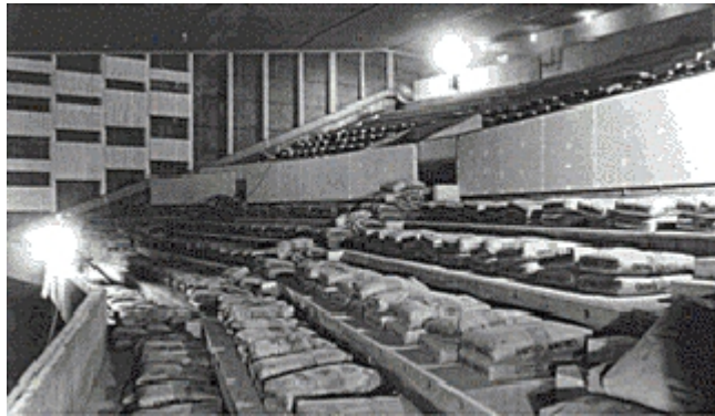
Load testing the circle at the Odeon , Marble Arch during construction
