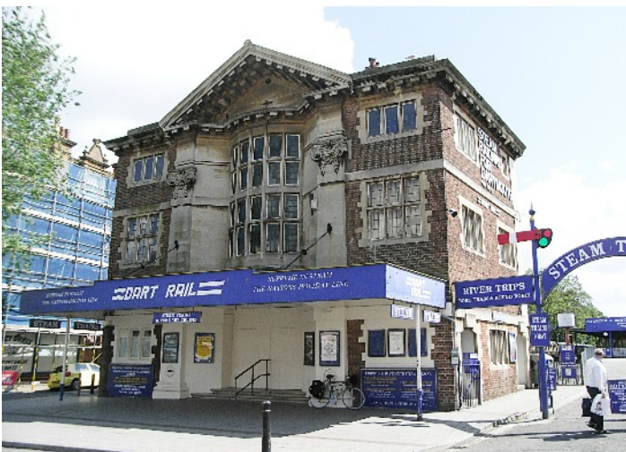
The Picture House Paignton in June 2008
