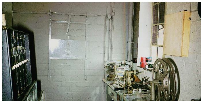
The rewind room at the Granada Rugby showing the fire shutters
