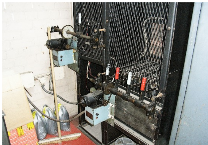
The main dimmer board at Sutton Coldfield
